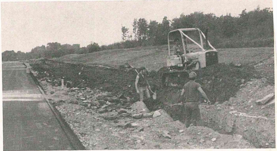
Backfilling of a trench that contains cable for the underground runway lighting system is accomplished with the use of a John Deere Model 450 dozer.
