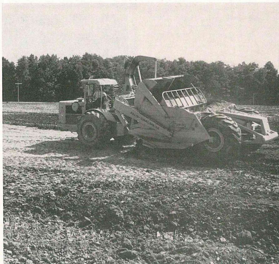
Spreading a thin lift, one of the seven Allis-Chalmers Model 260 scrapers saves time aerating and compacting the fill.
