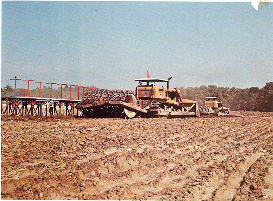
Drawn by an Allis-Chalmers Model HD-21 tractor, a 10-ft. wide sheepfoot roller compacts a lift. A Bomag Pack-All Model KB-4 steel-wheeled compactor works an adjacent section.
