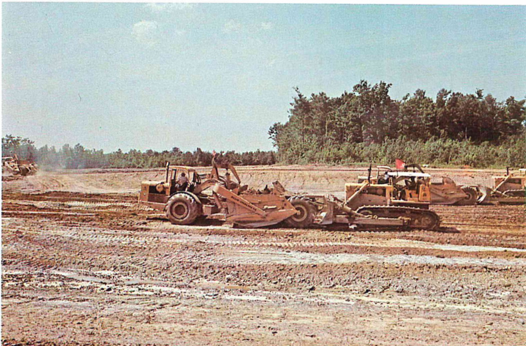
An International Model TD-25 tractor and an Allis-Chalmers Model 260 Series A scraper combine to excavate glacial till. Most of the material was hauled to an embankment for a future runway.
